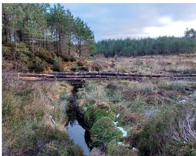
Leaky dams installation as a form of Natural Flood Management structure in Scotland.
